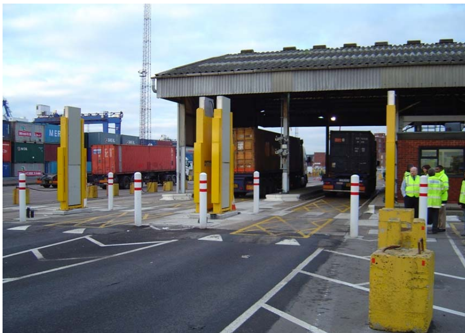
Figure 2. Radiation Portal Monitors in Felixstowe, U.K.
