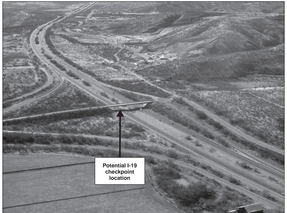
Figure 21: KP 25, Looking South, Aerial View, Location Marked
