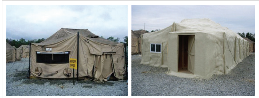
Figure 2: Tent before Application of Foam Insulation and Tent after Application of Foam Insulation
