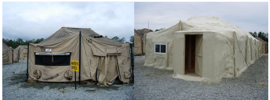
Figure: Tent before Application of Foam Insulation and Tent after Application of Foam Insulation
