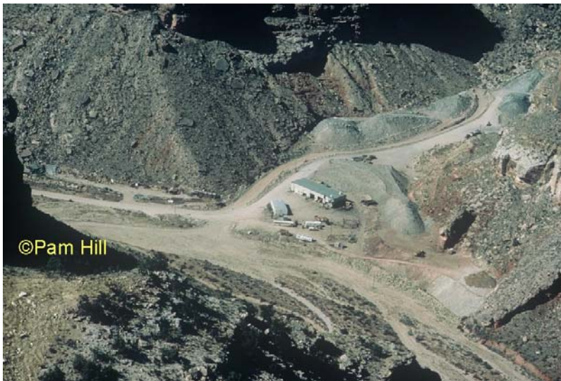
Figure 6. The Hack 1 Mine during mining (Hack Canyon, Arizona Strip). This was an underground mine that was in production during the 1980s. Note how little waste rock is sitting on the surface even during mining. As mining is closing the waste rock is backfilled into the drifts and stopes. Photo taken June, 1985 and courtesy of Pam Hill.
