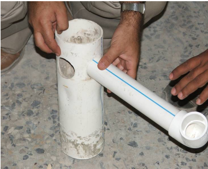
Site Photo 14. Typical contractor built wastewater pipe connection method
