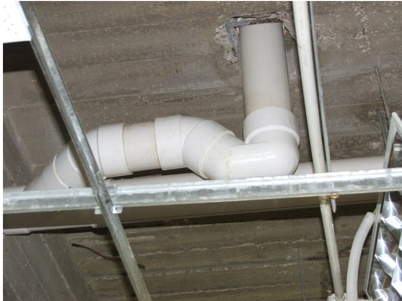
Site Photo 22. New pipe installed to correct the leak
