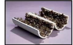
Clogged water pipe
