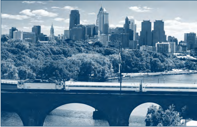
Regional | Schuylkill River Bridge, Philadelphia, PA
