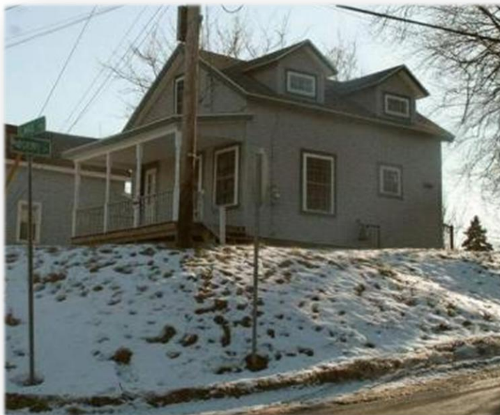
This house cost $105,000 to renovate, but was sold for only $42,000. The city neglected to survey the property prior to the renovation and as a result a driveway could not be added because the house is located on a steep hill.
