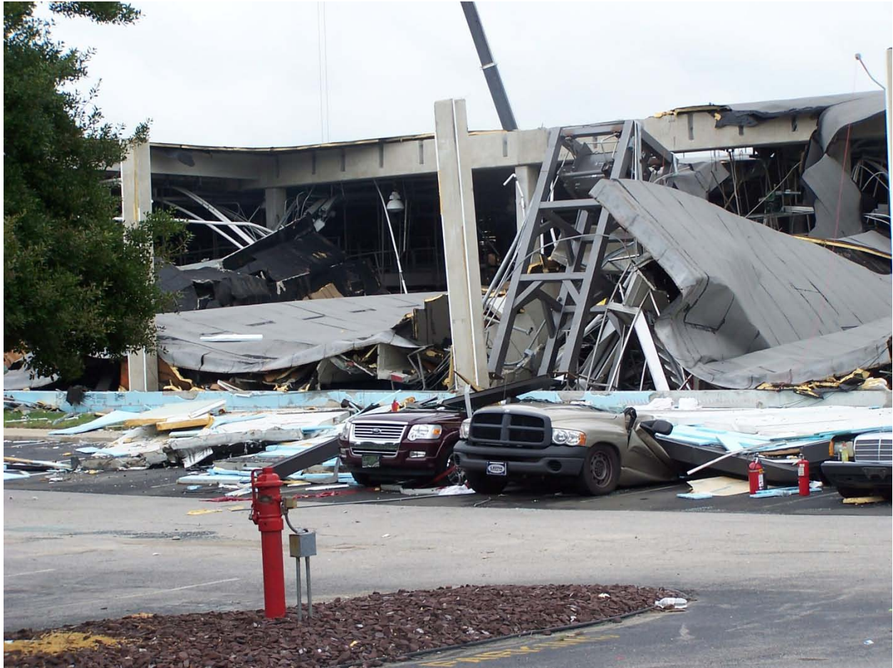
Figure 2. ConAgra Slim Jim meat processing plant in Garner, North Carolina, following the natural gas explosion of June 9, 2009, which killed 4 workers, injured 67 others, and caused much of the building to collapse.
