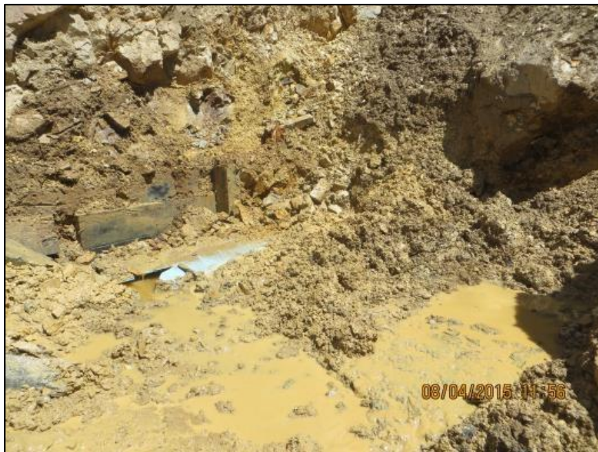
Photograph Showing Lower 24" Turquoise Drainage Pipe
