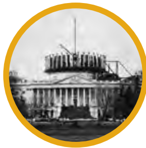
Construction of the Dome
