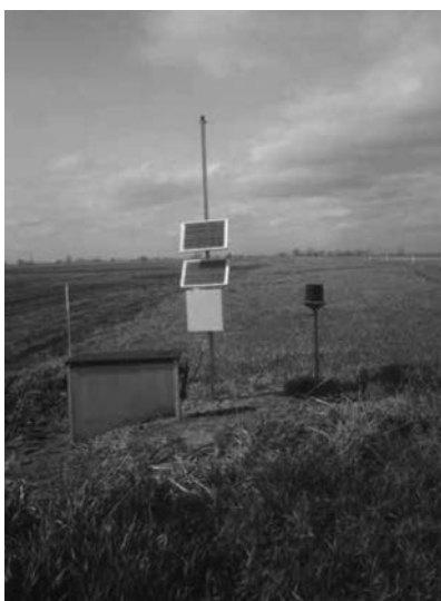
Automated instrumented DWM site—note how little land is taken out of production.
