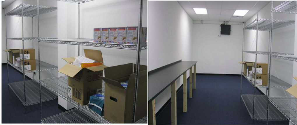
Figure VIII –Photos of LTC Pharmacy Taken by North Carolina Board of Pharmacy Inspectors
