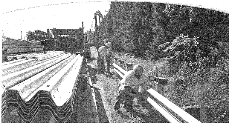
Installing guardrails to improve safety was a goal of several recovery projects.
