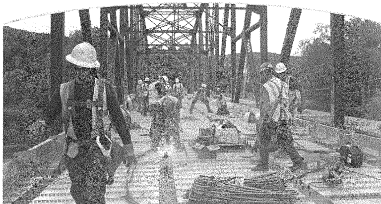
Workers on the Richmond, Vermont, bridge rehabilitation project.
