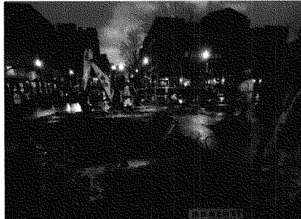
In this now iconic image which hangs in the Mayor's office lobby, City water crews work on a major water main break in the middle of Downtown Syracuse in February, 2013. (Credit: Anatoli Photograffi)
