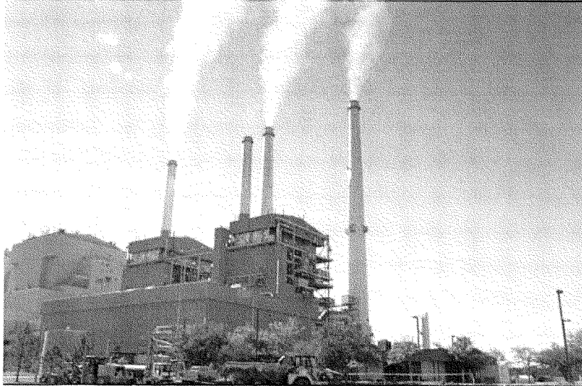
Smoke rises from the Colstrip Steam Electric Station, a coal-burning power plant in in Colstrip, Mont.
