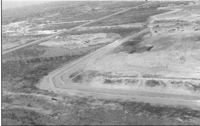
Picture B Old Gentilly landfill showing impact on cypress swamp and additional landfills 16 February 2007
