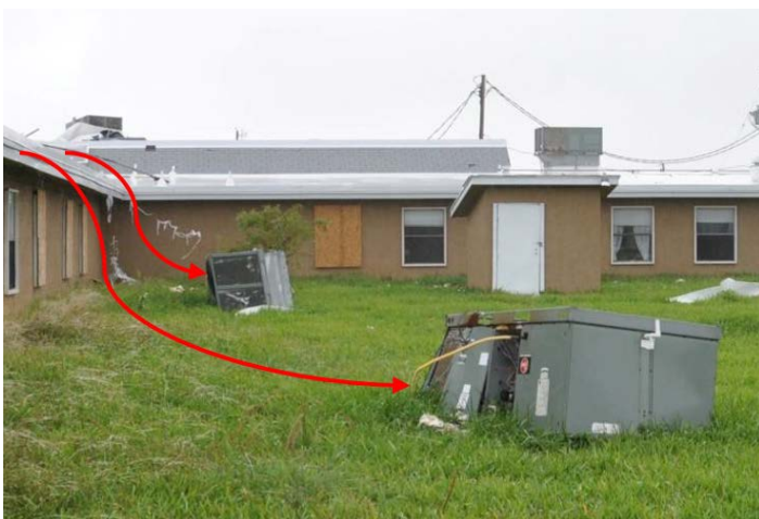
Figure 2. HVAC units at this nursing home were blown completely off the roof. Hurricane Harvey, Texas.
