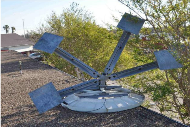
Figure 16. The satellite dish at this hospital was ballasted with concrete masonry units. The dish was nearly blown off the roof. Hurricane Harvey, Texas.
