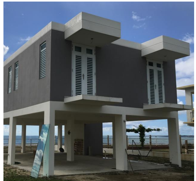
Figure 12. A well-built coastal structure with its lowest member above the BFE.
