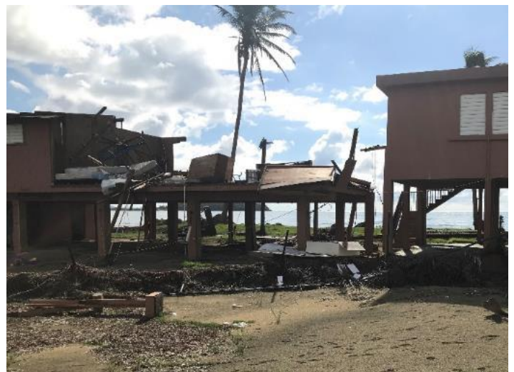
Figure 10. Structure foundation survived but could not resist high winds.
