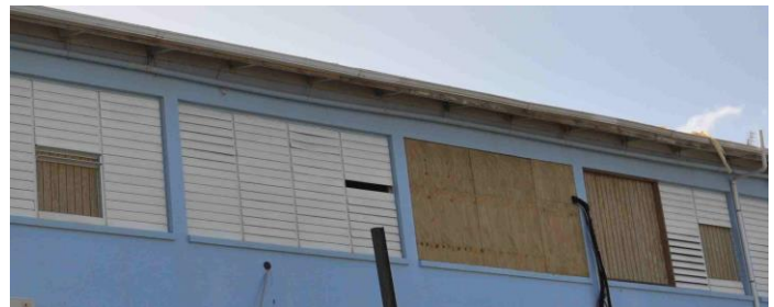
Figure 4. Several of the metal jalousie louvers at this school were blown away.
