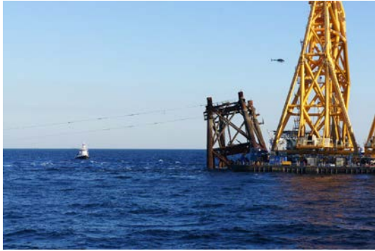
Jackets from decommissioned oil and gas platforms being deployed as artificial reefs off the coast of Louisiana
