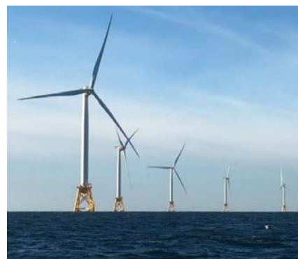
Block Island Wind Farm
