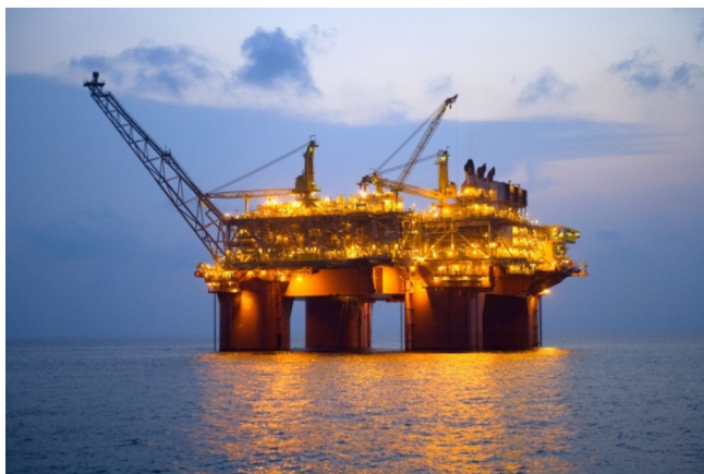
The Atlantis platform in the Gulf of Mexico
