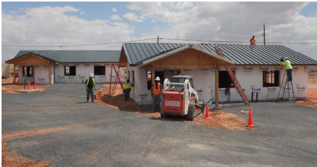
Moencopi Quarters under Construction
