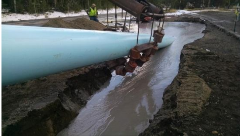
A section of new pipe is being monitored as it is placed (or replaced) as part of the Fishing Bridge waterline rehabilitation
