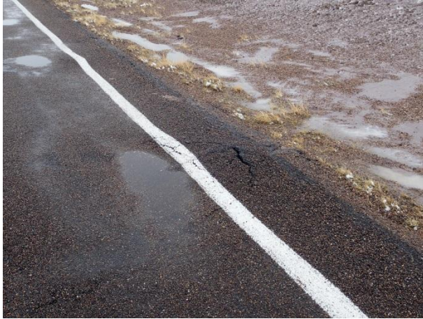
Pothole Repair in Petrified Forest NP.
