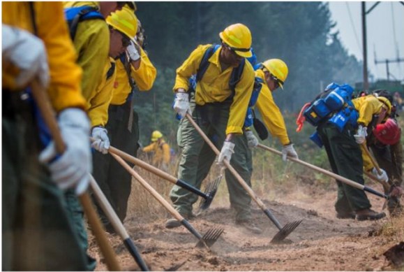
U.S. Army Soldiers, assigned to 23rd Brigade Engineer Battalion, 1-2 Stryker Brigade Combat Team, complete initial tactical training with the BLM's Devils Canyon Veteran Crew, Umpqua North Complex, Oregon, Sept. 8. The soldiers learned how to construct a fireline, which is made using hand tools to cut, scrape or dig to remove brush and debris that might fuel the spread of the fire. (Photo by Pvt. Adeline Witherspoon, 20th Public Affairs Detachment)
