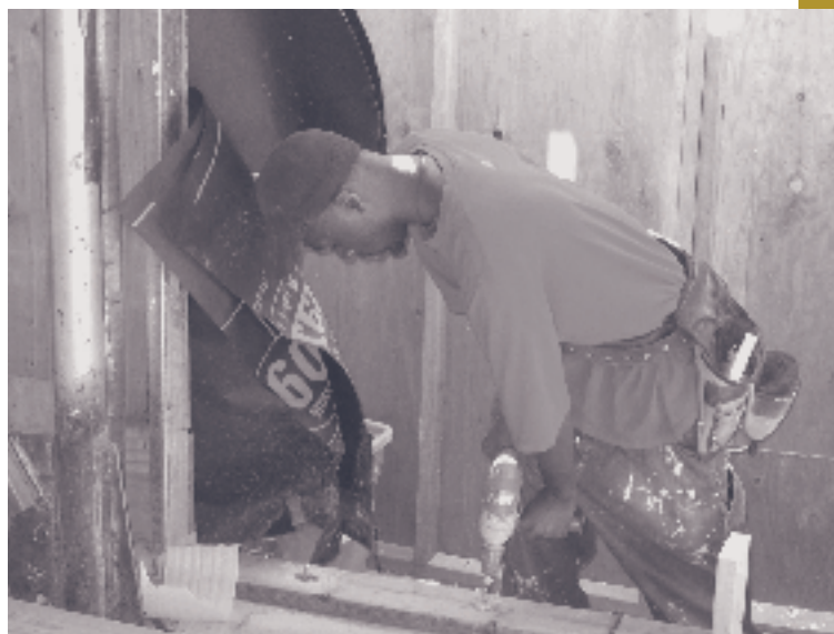
A YouthBuild student works on the YEP building.
