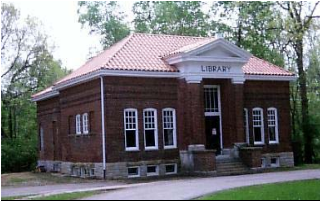
The Lawrie Library, after rehabilitation work— DNR Division of Historic Preservation and Archeology
