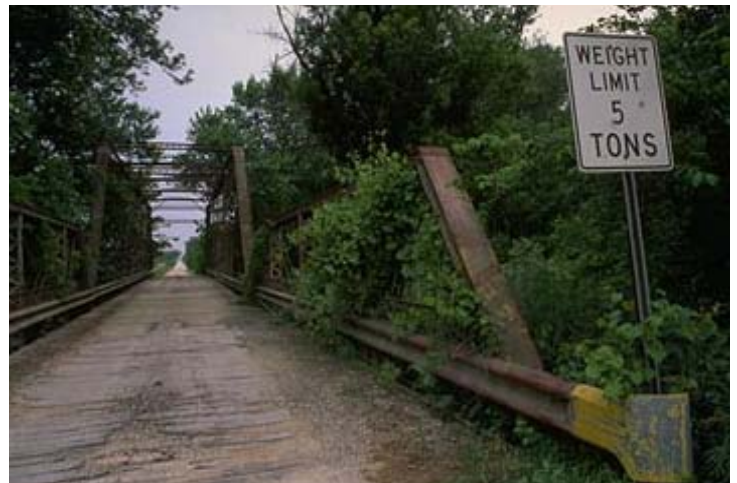
1st Wabash River Bridge- Richard Fields
