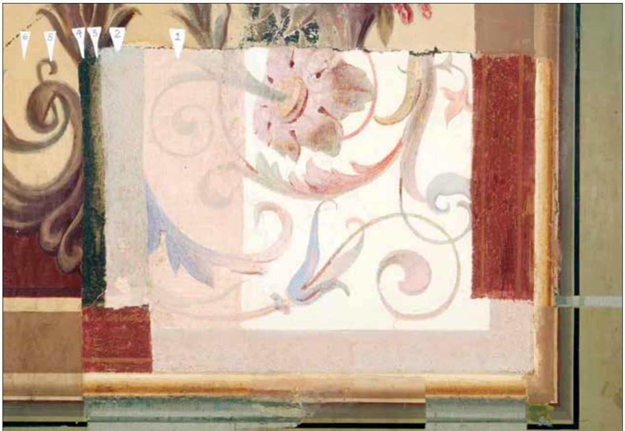
Overpaint altered the appearance of the murals in the Brumidi Corridors. Numbered arrows indicate the six layers of overpaint applied successively over a century to the original surface.
