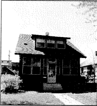
739 Curfew Street, looking west
