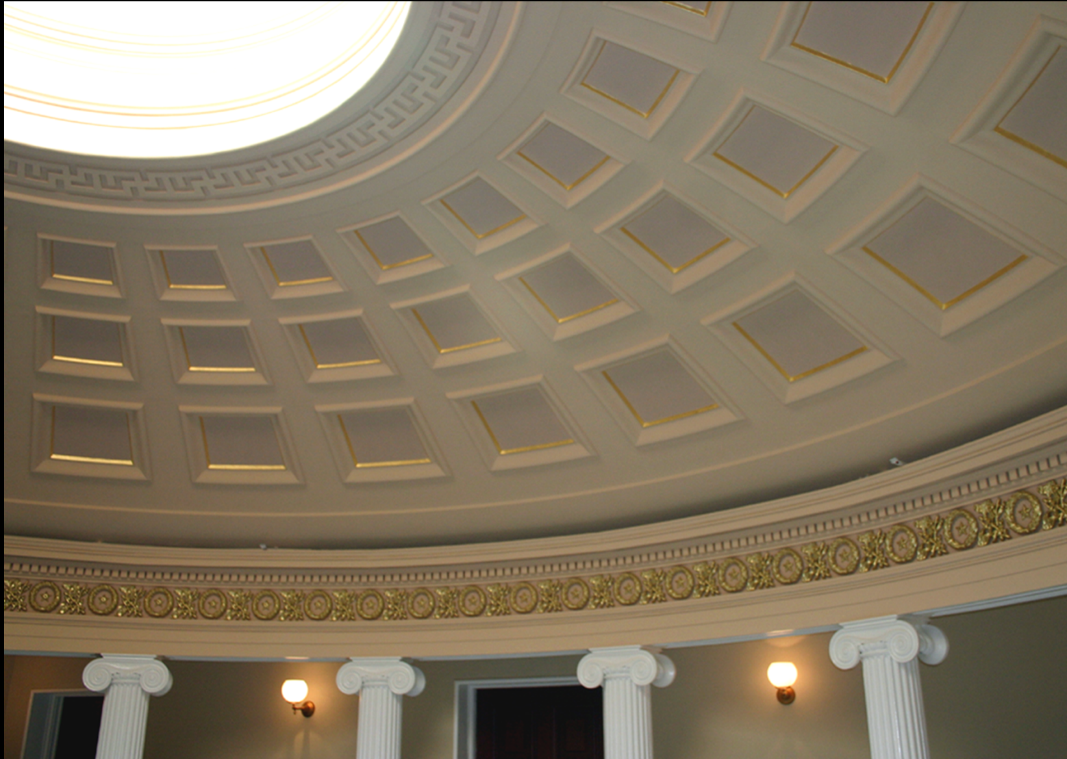
Completed Restoration of the Southwest Dome
