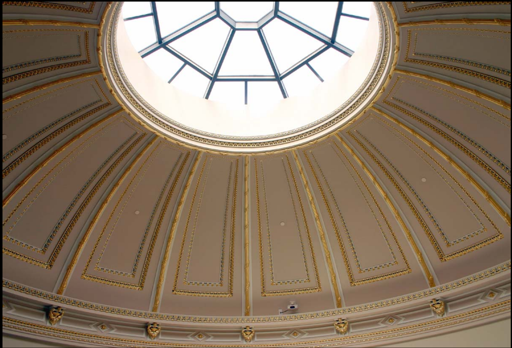
Completed Restoration of the Northeast Dome
