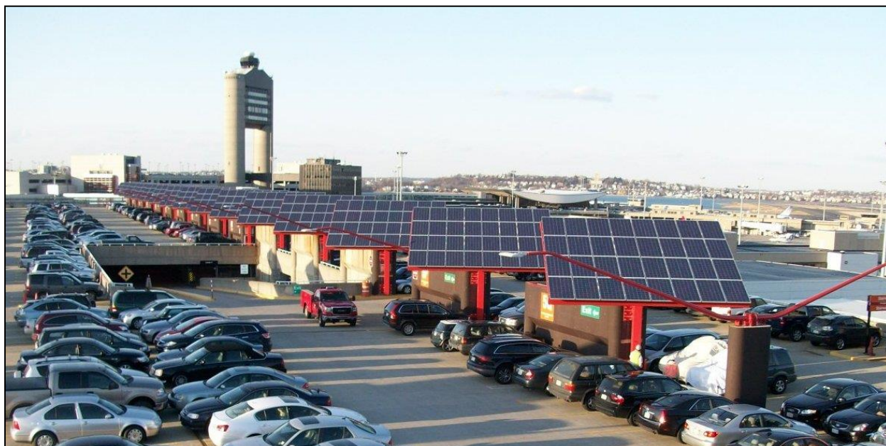
Figure 20: Solar Trees on Parking Garage at Boston’s Logan Airport
