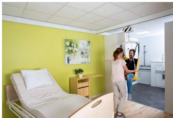
Figure 7. Overhead lift on traverse track system covering both bedroom and bathroom, with traveling rail moving through a gap in the separating wall. Photo Courtesy of Guldmann Inc.™ Reprinted with Permission – All Rights Reserved
