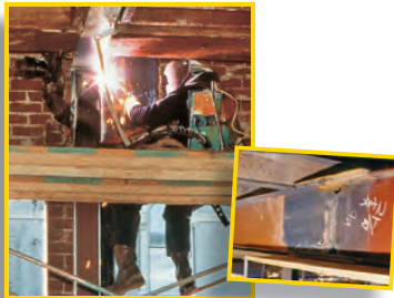
Strip back paint before cutting or welding.
