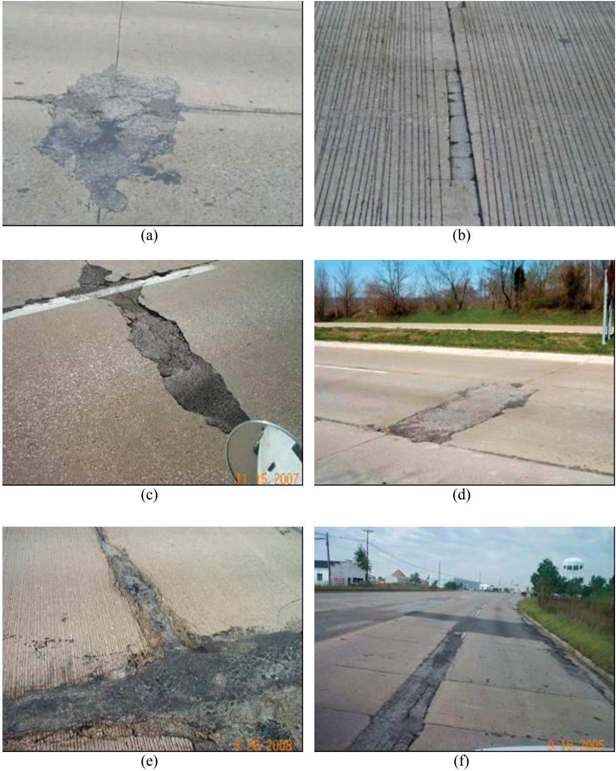
FIGURE 3-24 Patch/patch deterioration: (a) and (b) moderate severity; (c), (d), (e), and (f) high severity
