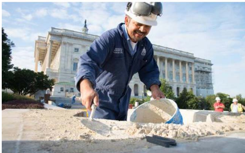
AOC stonemason makes repairs to the Olmsted Terrace Walls.
