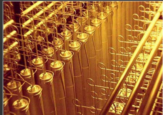
Bank of centrifuges Source: Urenco LTD.
