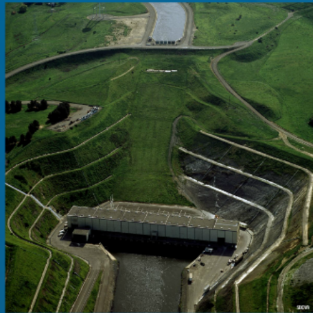
Harvey O. Banks Pumping Plant
