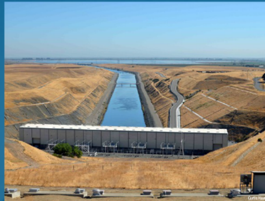
C.W. "Bill" Jones Pumping Plant
