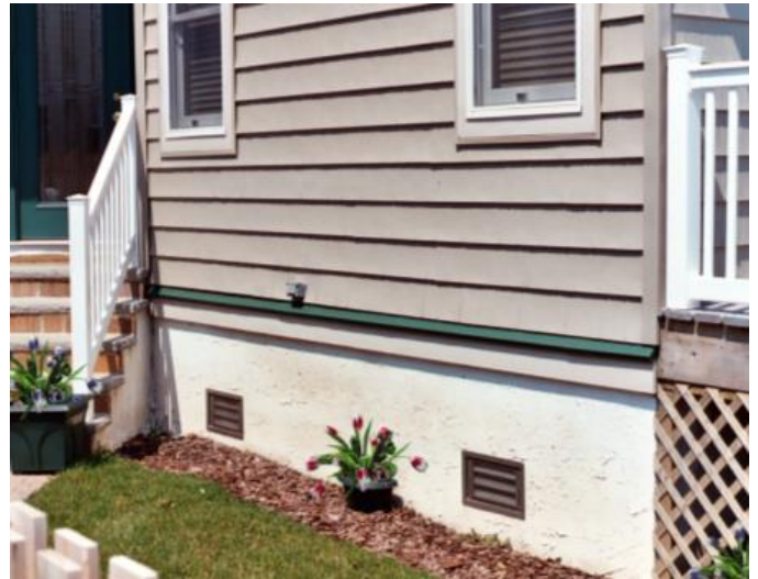
Figure 6. Example of hydrostatic openings (red circles). From FEMA TB-1 (cover image).
