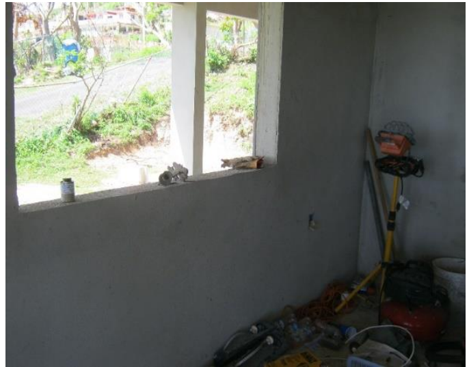
Figure 3. Typical concrete interior finishes on a residence under construction in Yabucoa.
