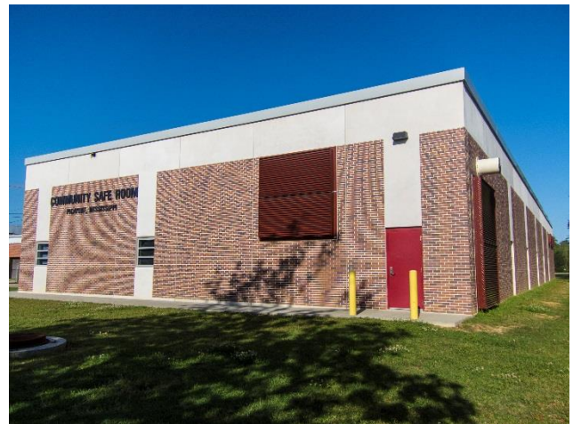
Figure 1. FEMA funding was used to construct this safe room at Picayune High School, Picayune, Mississippi. As part of the Mississippi Post-Katrina Safe Room Initiative, it was constructed with financial assistance from the FEMA Hazard Mitigation Grant Program (HMGP).
