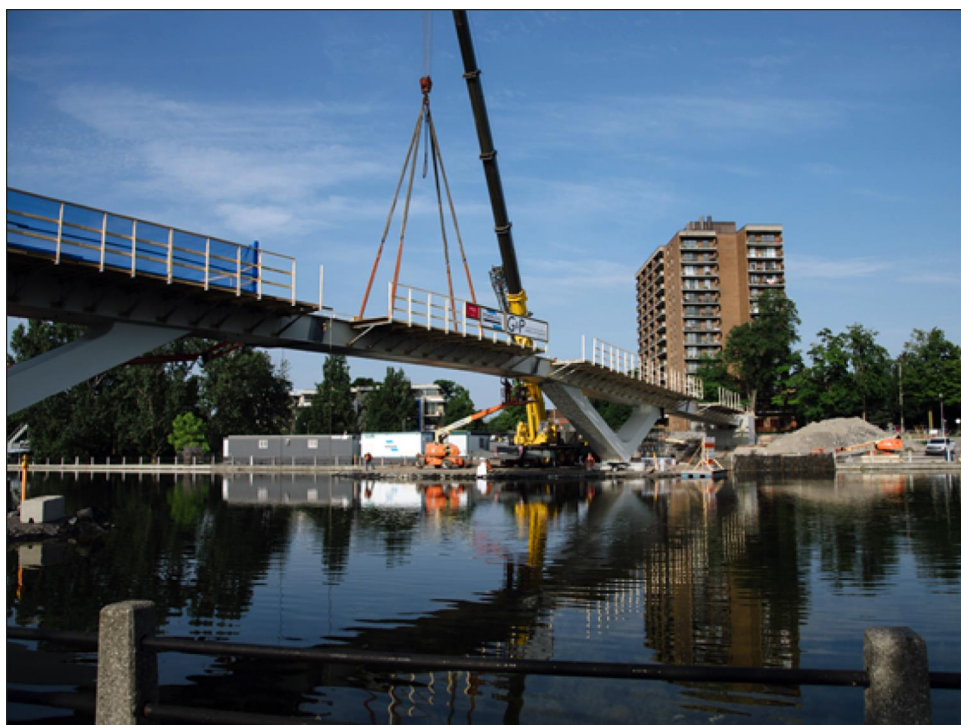
Figure 7: Flora Footbridge, Ottawa, Ontario Canada
