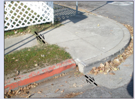
Creep (slow, steady movement) on the Hayward Fault has offset this curb in the city of Hayward.
