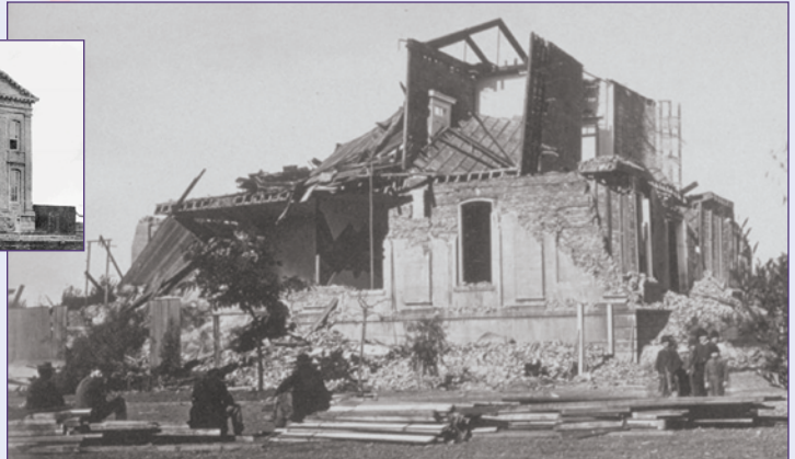
Strong shaking during the 1868 Hayward Fault earthquake caused the second story of the Alameda County Courthouse in San Leandro to collapse (photo courtesy of the Bancroft Library, University of California). The inset photo shows the courthouse before the quake (photo courtesy of San Leandro Public Library). The 1868 earthquake devastated several East Bay towns and caused widespread damage in the San Francisco Bay region.
