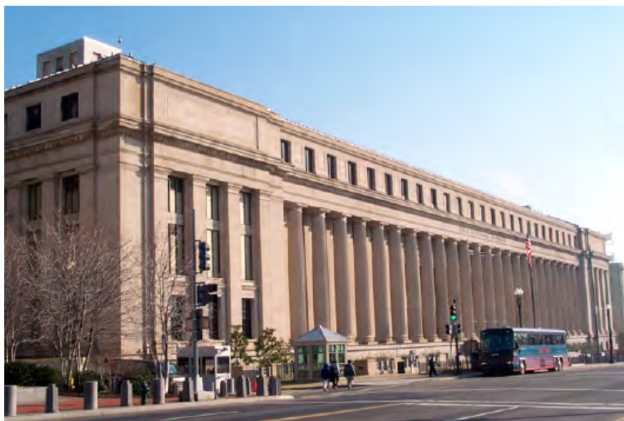
Treasury’s ownership of some buildings creates a different set of concerns than managing leased space.
