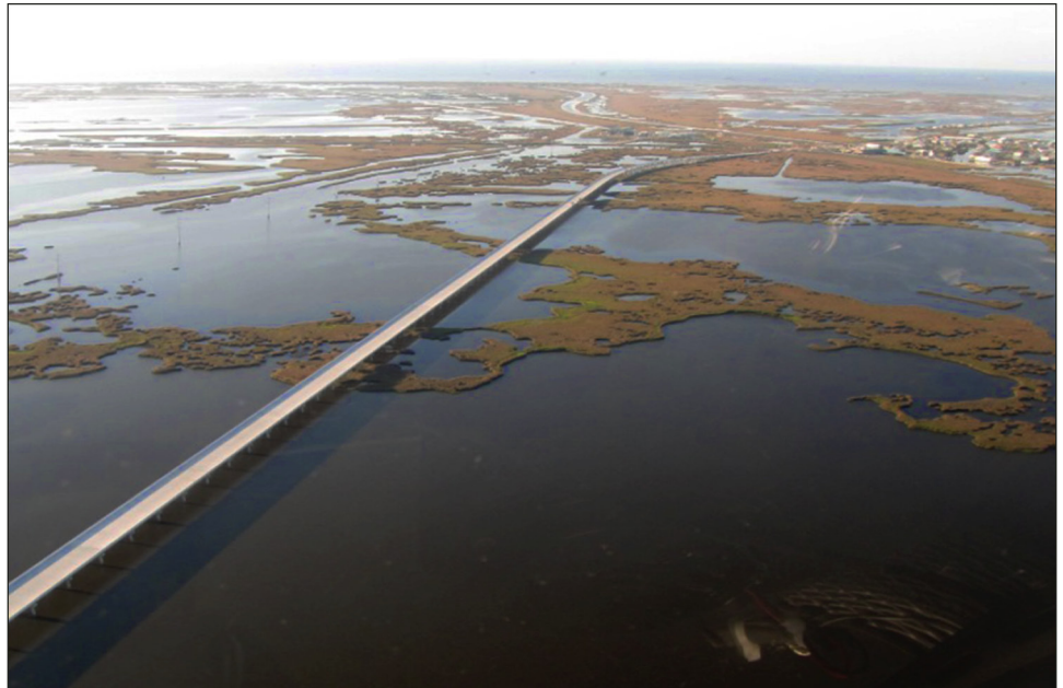
Figure 4: Louisiana State Highway 1 Leading to Port Fourchon
