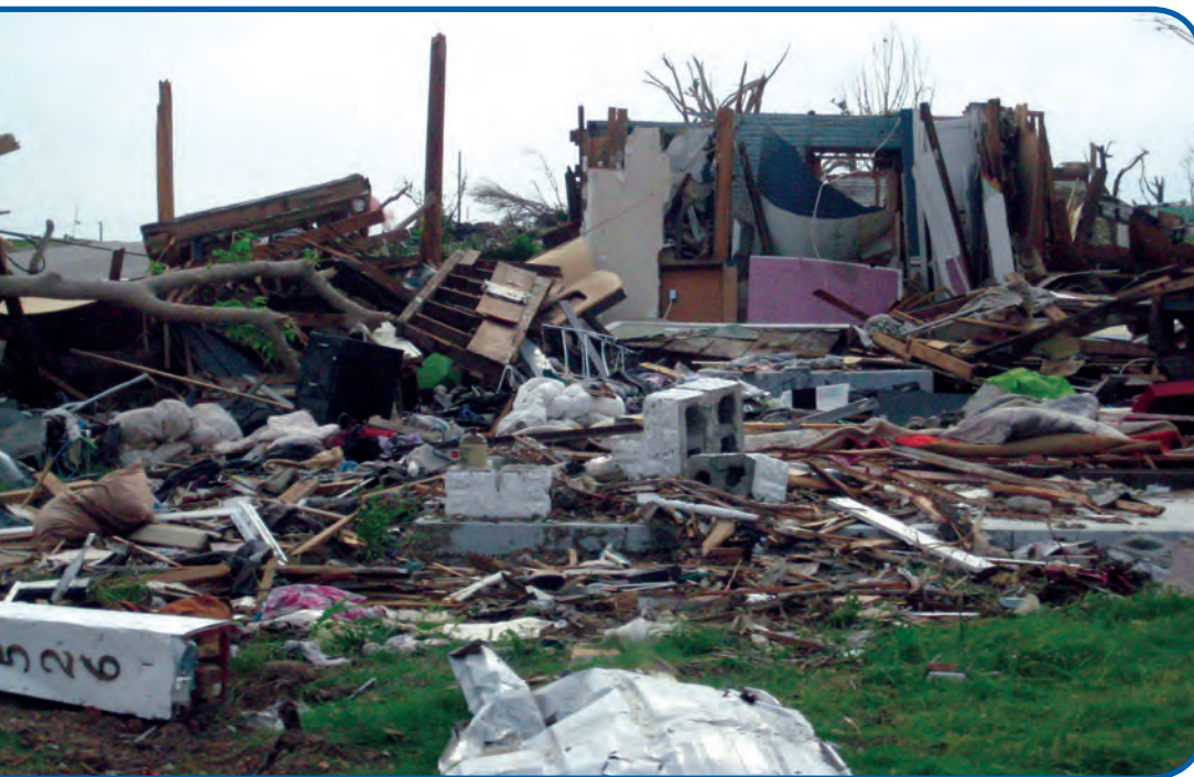
▲ This photo, taken approximately 5 weeks after the tornado, shows the remains of a mucormycosis case-patient's home that was destroyed.
