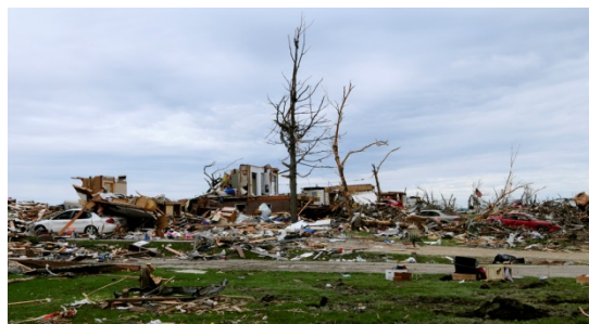
Figure 11. Debris on Private Property
