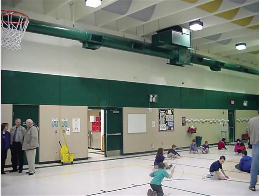
Figure A4-1. Example of a multi-purpose safe room also used as a gymnasium
