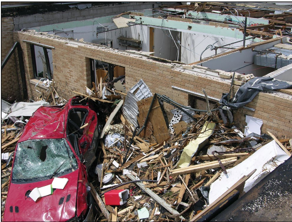
Figure B8-10. Representative quantity, size, and type of debris that is often generated by a strong or violent tornado. The building damage at this site was indicative of an EF3 tornado. (Greensburg, KS, 2007) (SOURCE: FEMA P-577)
