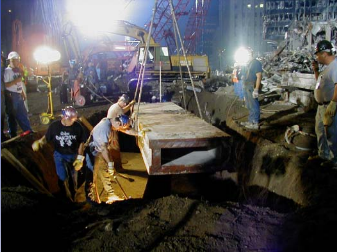
Clean weld fracture of Interior columns
