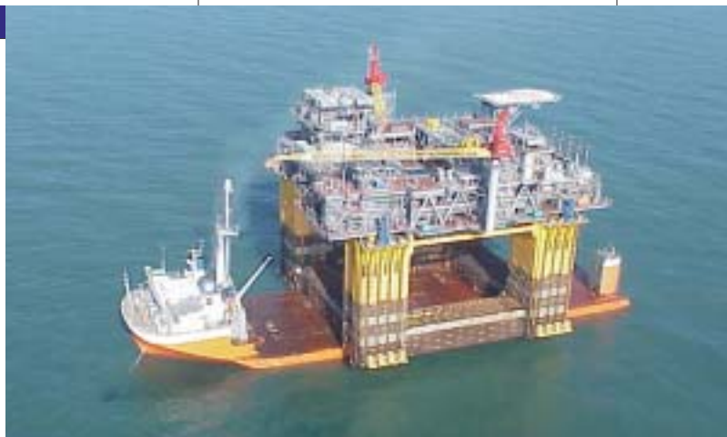
Above: Na Kika semisubmersible platform, all 40,000 tons, being transported offshore. Photo courtesy of BP Exploration & Production Inc.
