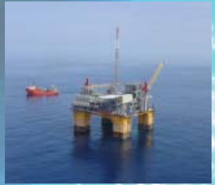
Na Kika in the Gulf of Mexico. Photo courtesy of BP Exploration & Production.
