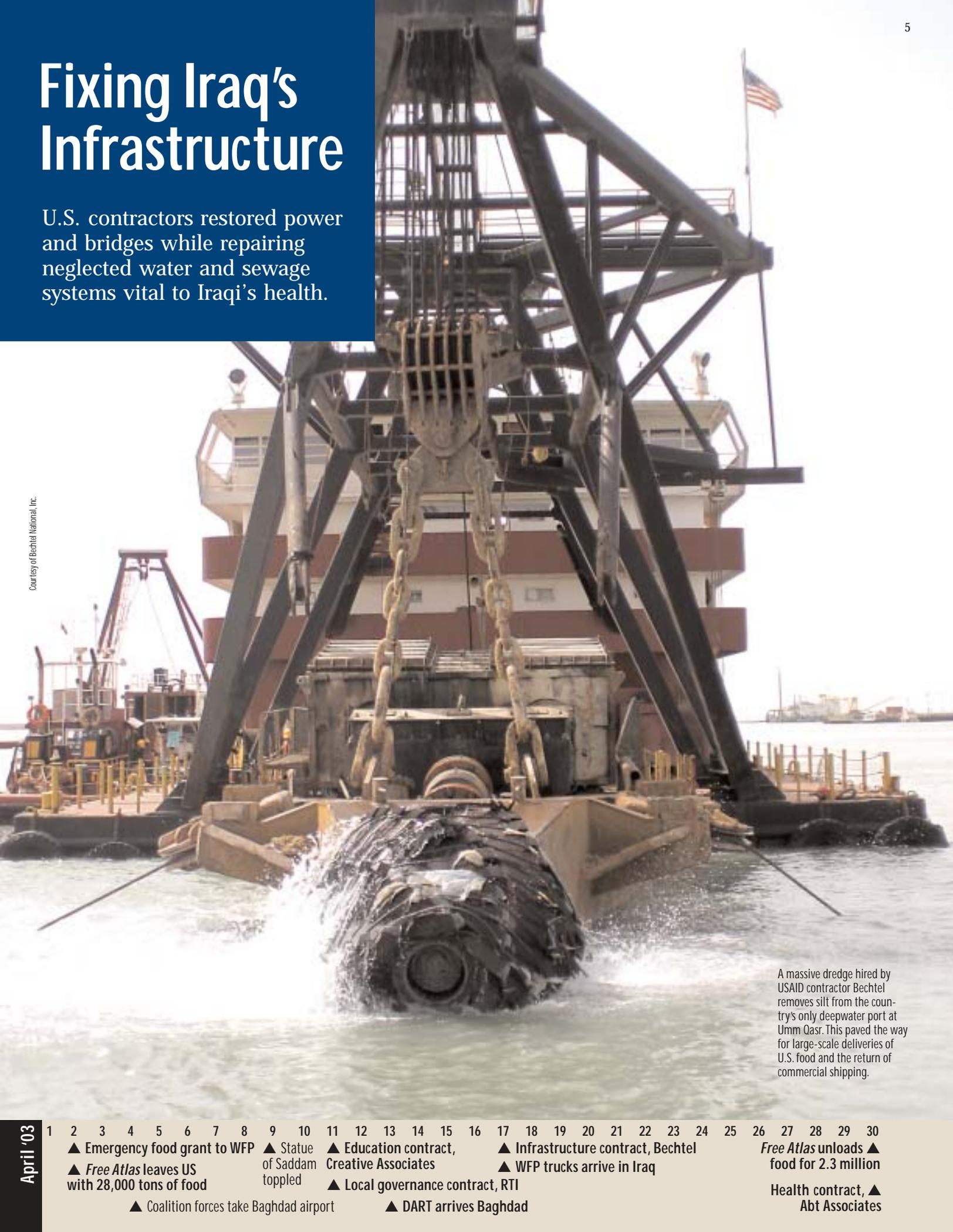
A massive dredge hired by USAID contractor Bechtel removes silt from the country's only deepwater port at Umm Qasr. This paved the way for large-scale deliveries of U.S. food and the return of commercial shipping.
