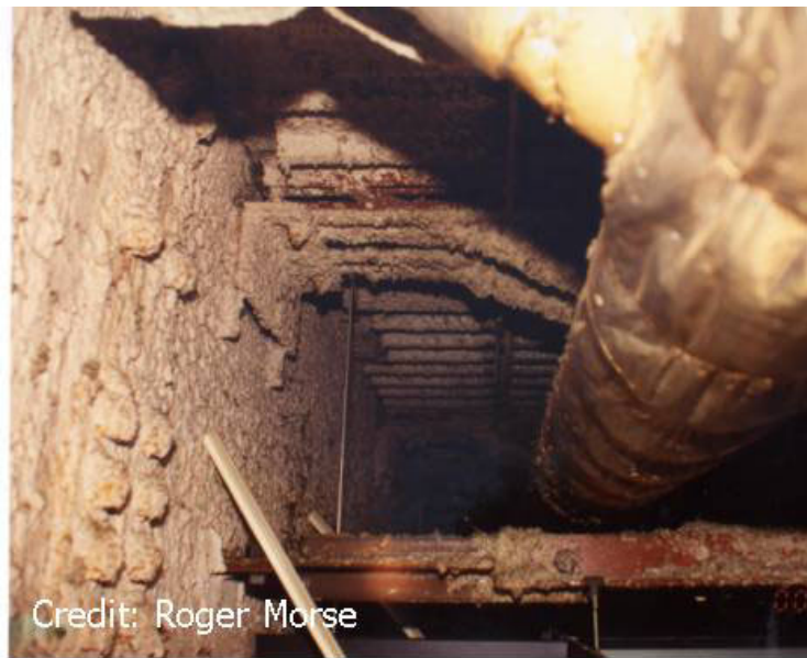
Figure 10. Missing spray-on fire proofing around a connection (left ) and missing fireproofing panels on a steel column (Mowrer).
