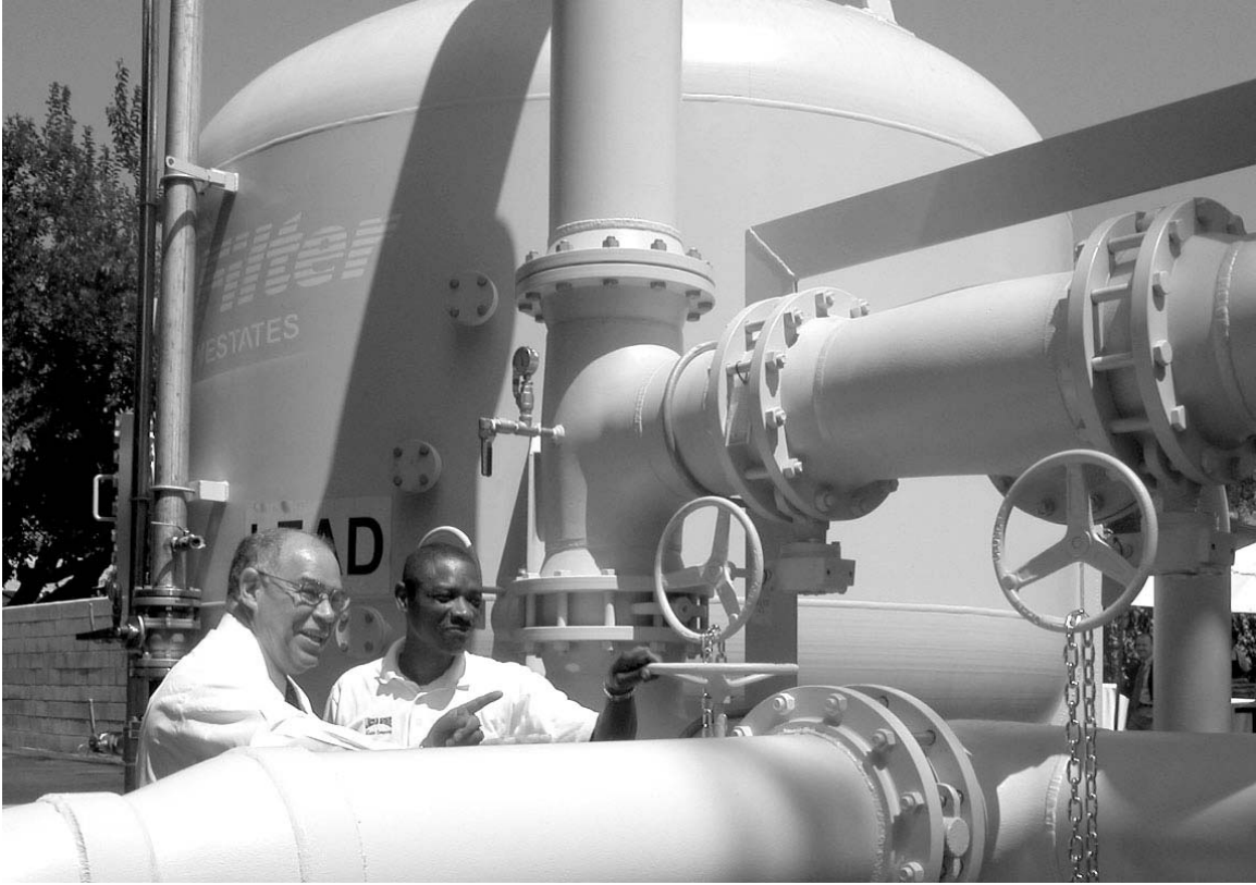
NASA's Deputy Administrator Fred Gregory (left) and LAWC's General Manager Bob Hayward (right), recently launched LAWC's Ion Exchange System to remove perchlorate from groundwater.
